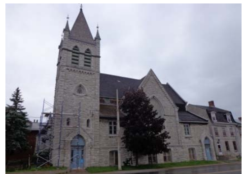
Ongoing alteration work-former Queen Street United Church
