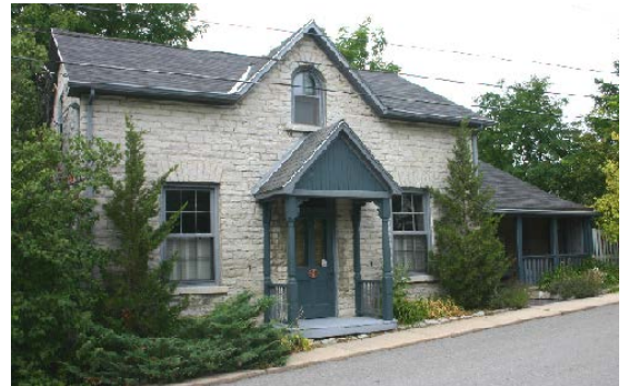
Compatible addition at the side of an 1850s limestone cottage, Barriefield Heritage Conservation District
