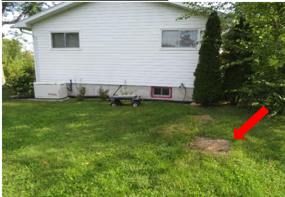
General tank location
