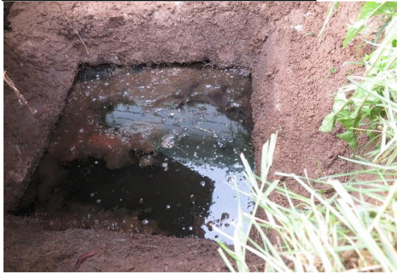
Liquid level in tank
