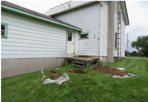
General tank location
