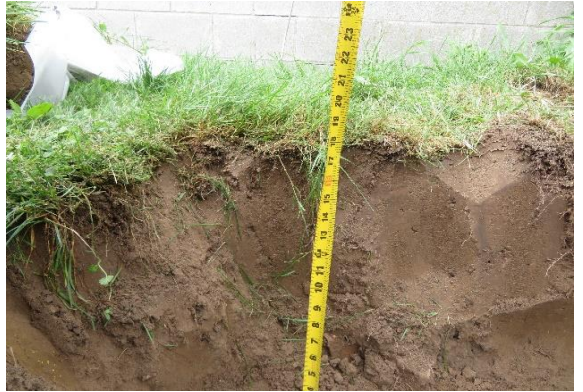
Depth to top of tank
